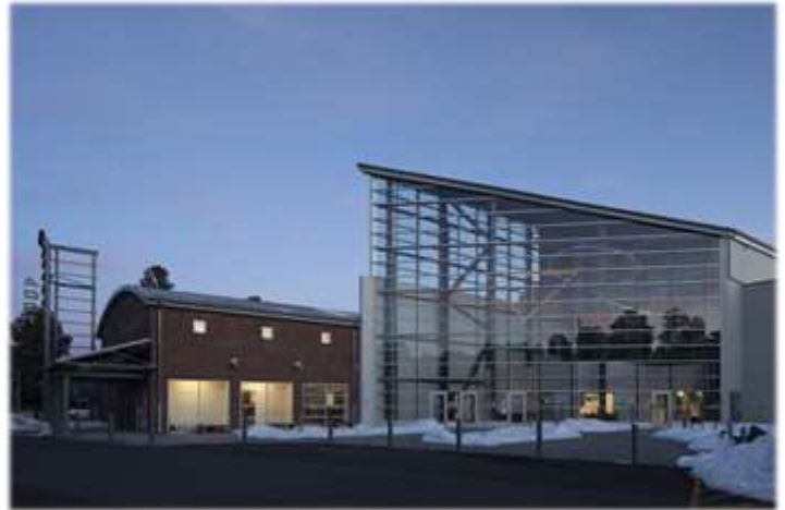
The Arizona Department of Transportation converted a 9-screen Harkins movie theater in Flagstaff into a 72,000 square foot, 2-story headquarters and office for the Motor Vehicles Division.
